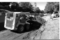
and remove excess sediment, while the slope will be stabilized by planting 4,000 trees and plants. The drainage conveyance system, along with fencing and filter screens, will control erosion along the river.
